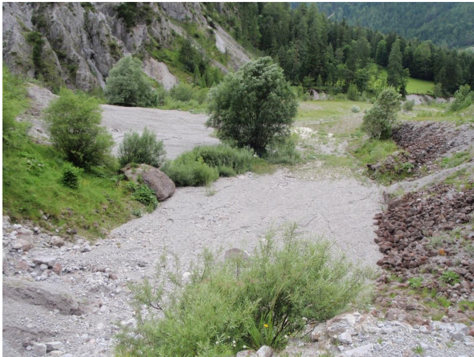
Figure 3: Situation in 2017 - mosses, willows and higher plants form a rich spring habitat - which is covered by gravel from both sides. Picture: C. Remschak, 2016
