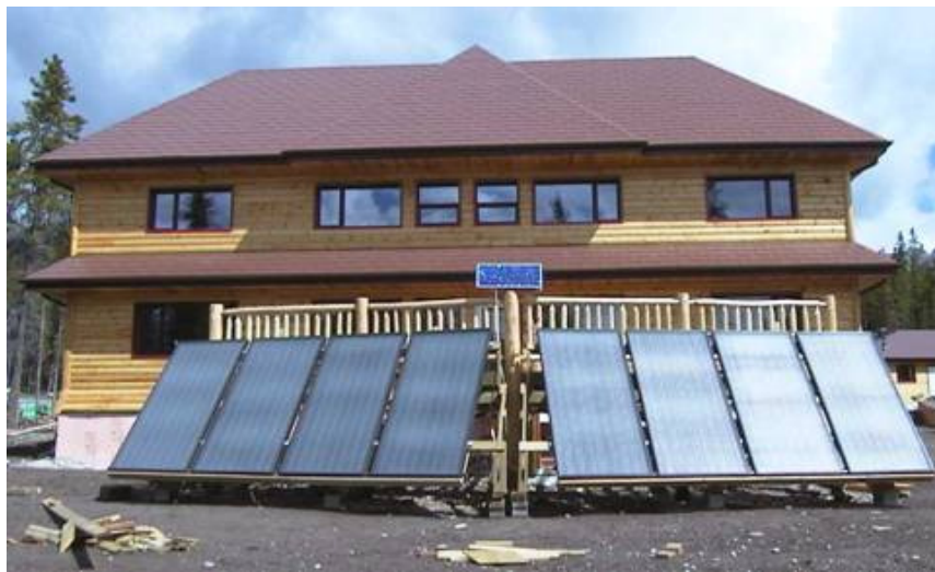
Figure 11 – Solar Collectors of Aurum Lodge, Alberta, Canada
