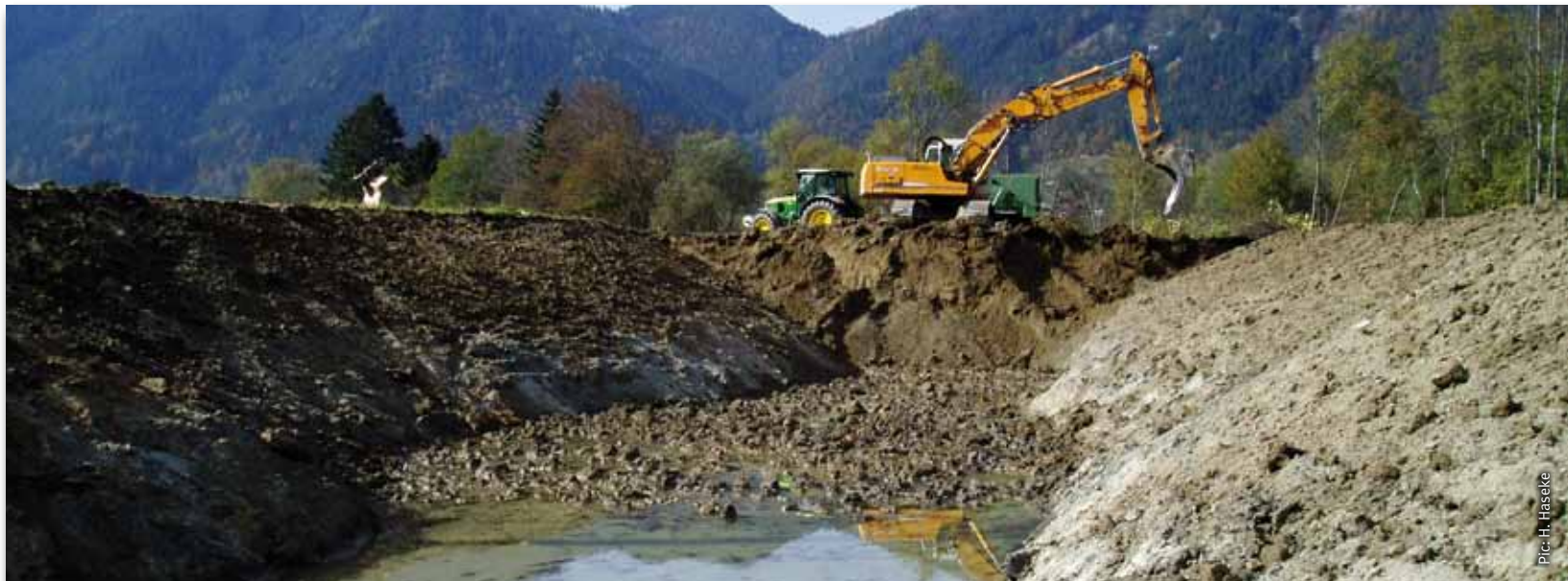
Digging of a new stream reach in October, 2006. All in all, we had to move more than 30.000 cubic metres of soil and sand.
