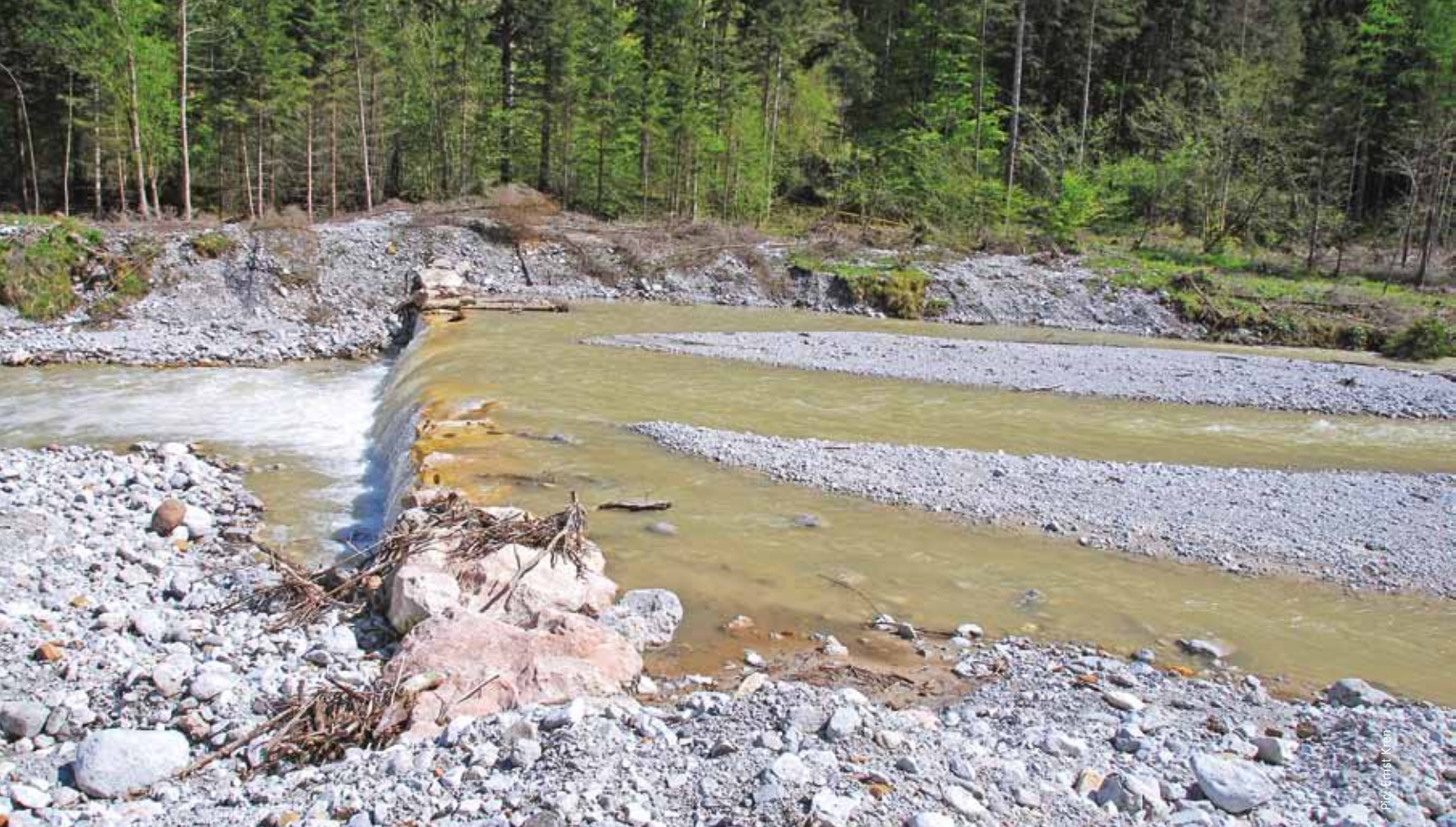
Several sills remain too high because of the lack of dynamic bedload and the erosion of the riverbed which had been disturbed during the construction phase. This might be a problem for weak fish like the brook lamprey.
