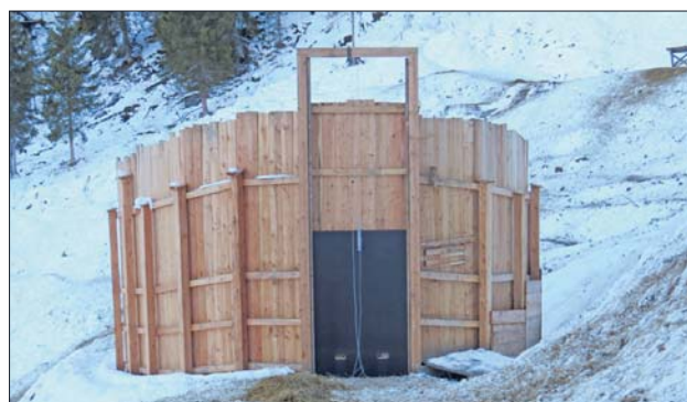
Construction of the capturing kraal in the National Park area of the Habach Valley. The interior is designed so that the red deer cannot injure themselves. The side walls are about four meters high. Wildlife enters through two openings in the kraal. The entrances can be closed again using trap doors.
